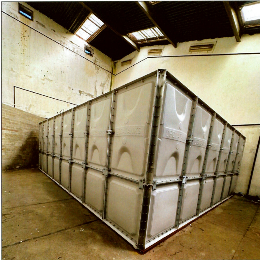
Figure 3.2: Water tank located within former handball court. (Source: IMAC Group, 2025).
