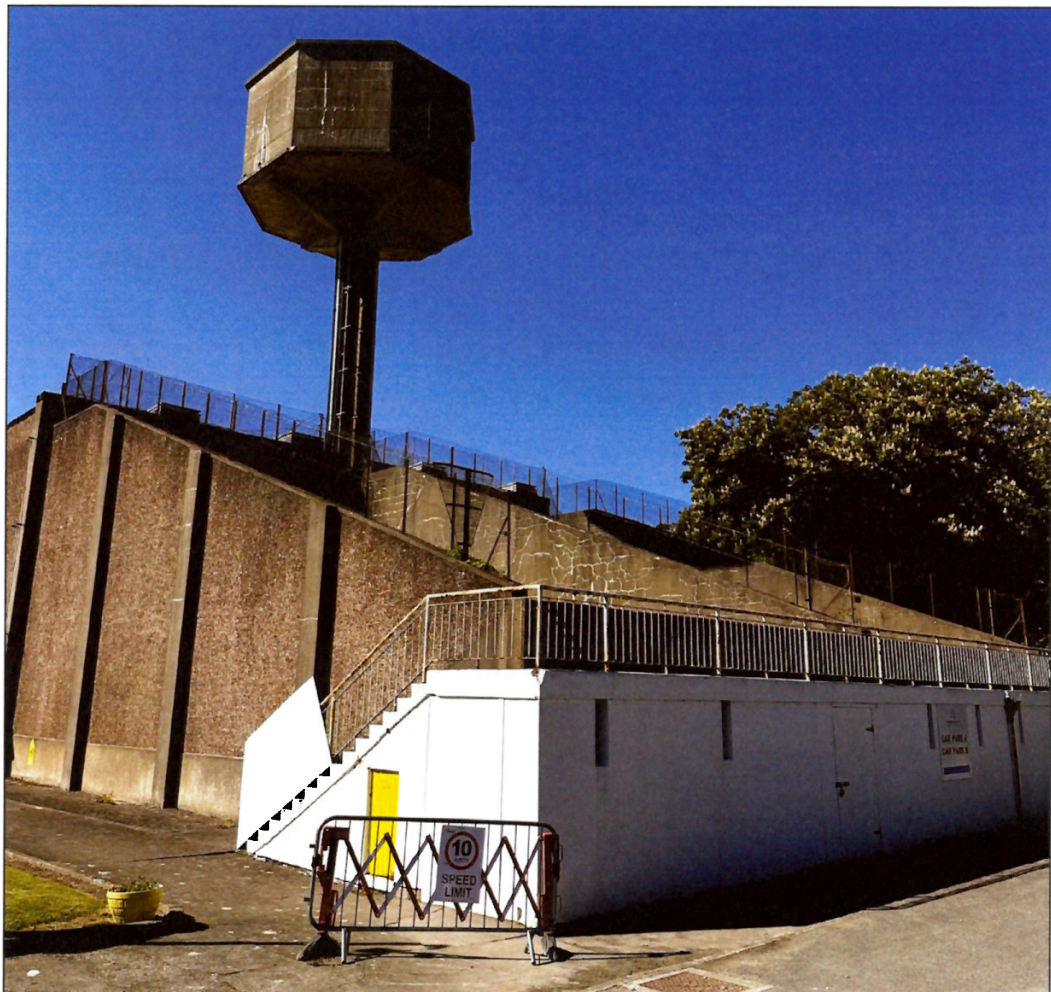
Figure 3.1: Disused handball alley and historic water tank. (Source: IMAC Group, 2025).
