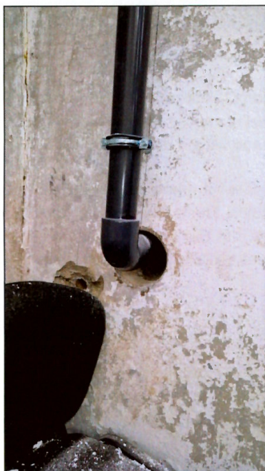
Figure 3.3 and Figure 3.4: Holes cored into walls of former handball courts. (Source: IMAC Group, 2025).
