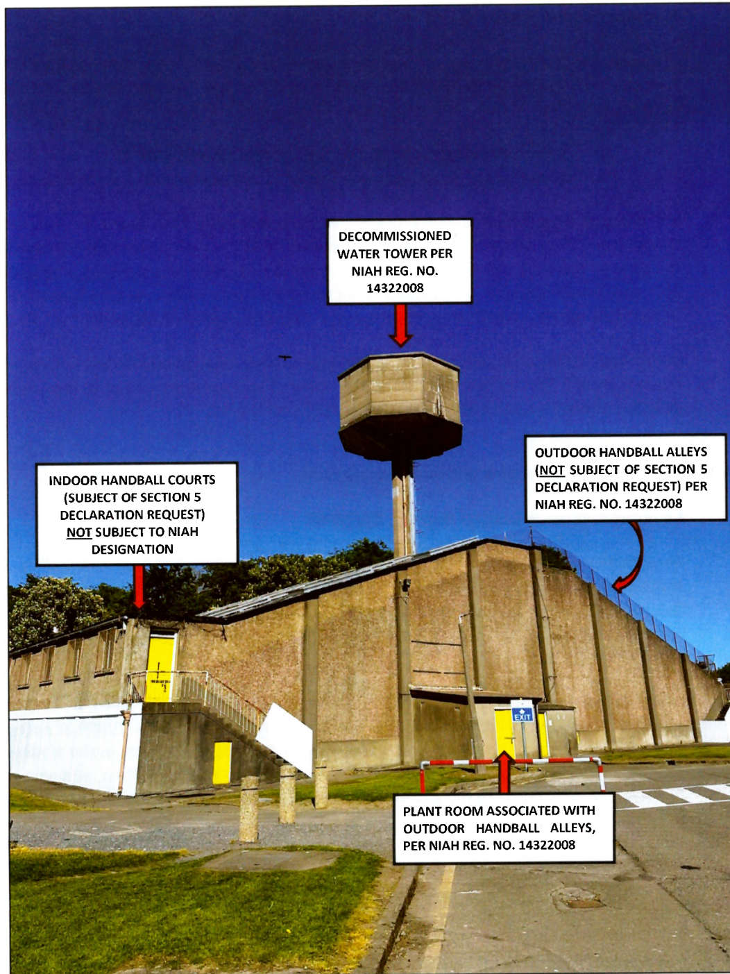
Figure 3.1: Image showing locations of indoor handball courts, versus outdoor handball alleys and associated plantroom and water tower. (Source: IMAC Group, cropped and annotated by TPA, 2025).
